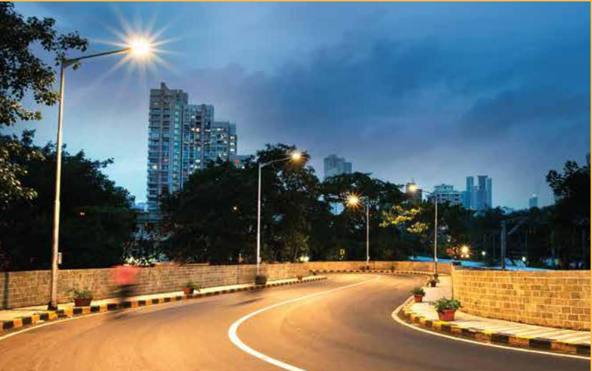
S Bridge Lower Parel, Mumbai
