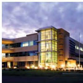
8 Facade and Exterior Lighting
